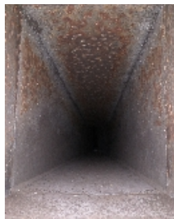
● CORROSION ●
